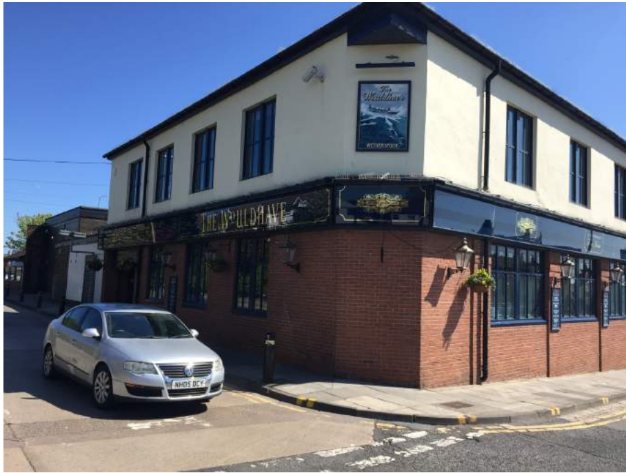
Existing The Wouldhave public house Viewed from corner of Mile End Road and Coston Drive
