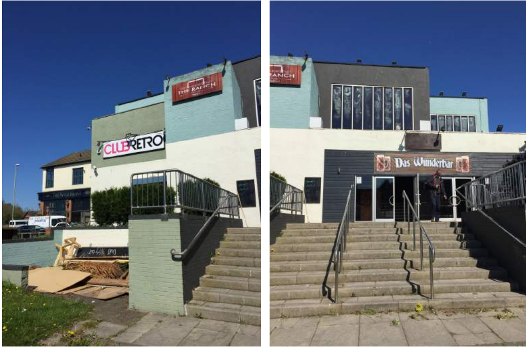
Existing vacant nightclub Viewed from the rear
